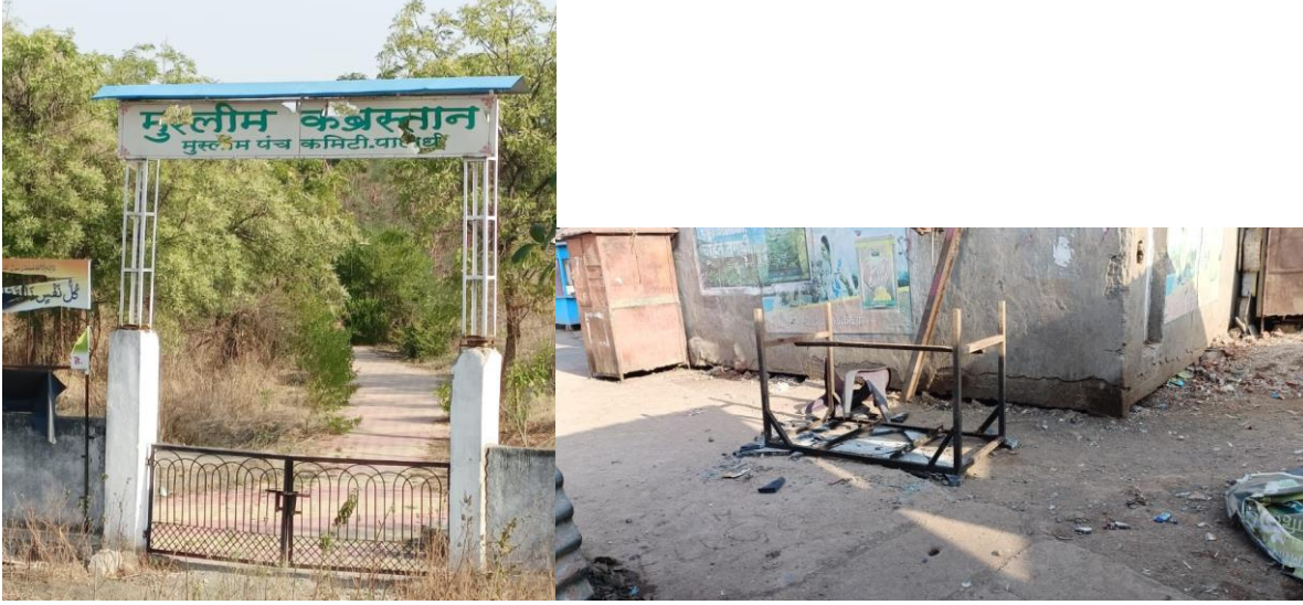
A damaged entrance of a Kabristan and ruins after the clashes in Paldhi
