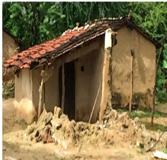
A Bhil house devastated due to the rains
